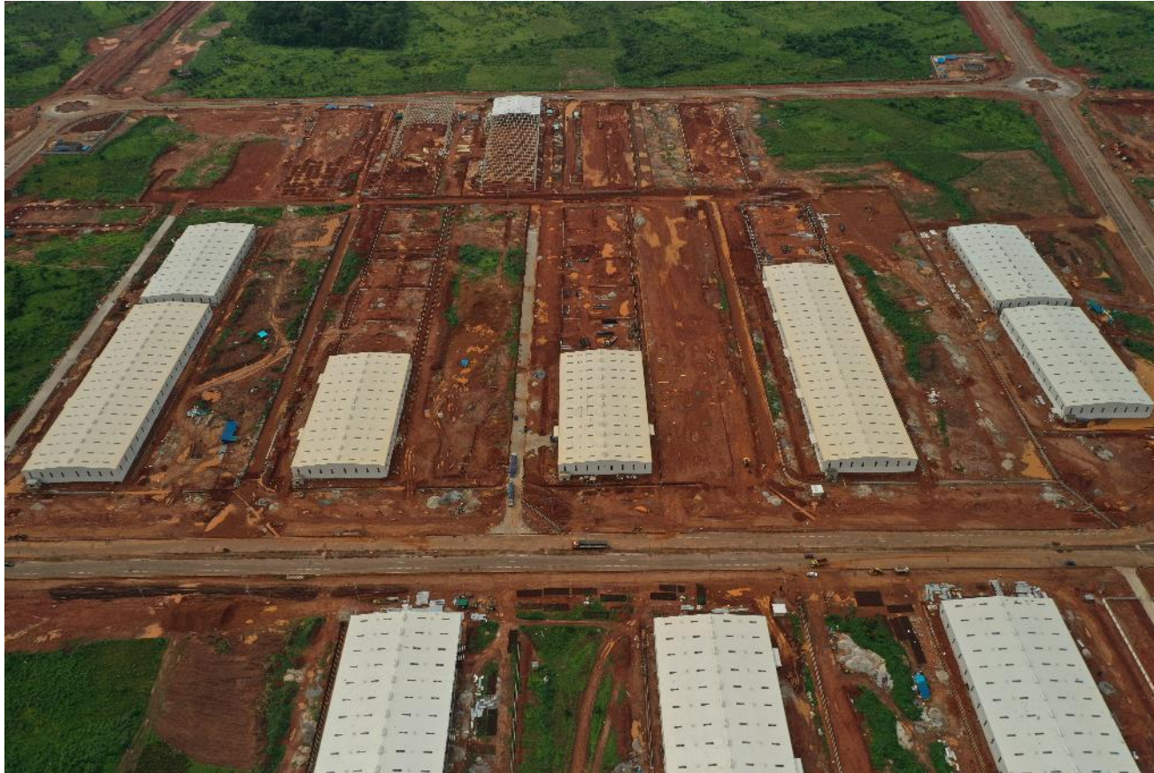
Warehouses under construction - GDIZ
